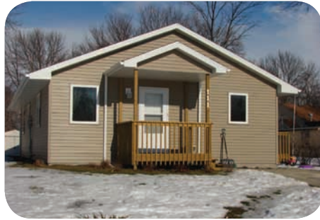
111 Park Street (November 2007)
